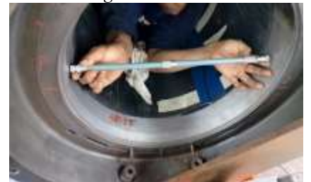
Fig 4. Checking the bearing's internal diameter after installation.
