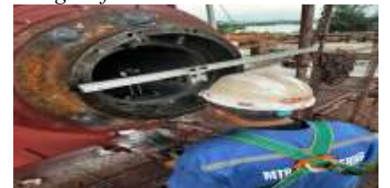
Fig 3. Alignment check after installation of the new bearing.
