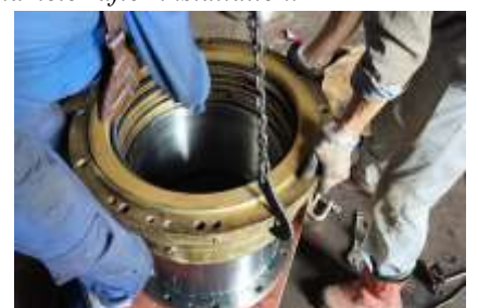
Fig 5. Seal installation at the workshop
